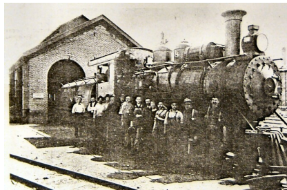
NCO Locomotive Shop and Crew
